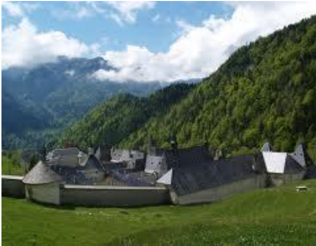
La Grande Chartreuse monastery near Grenoble
